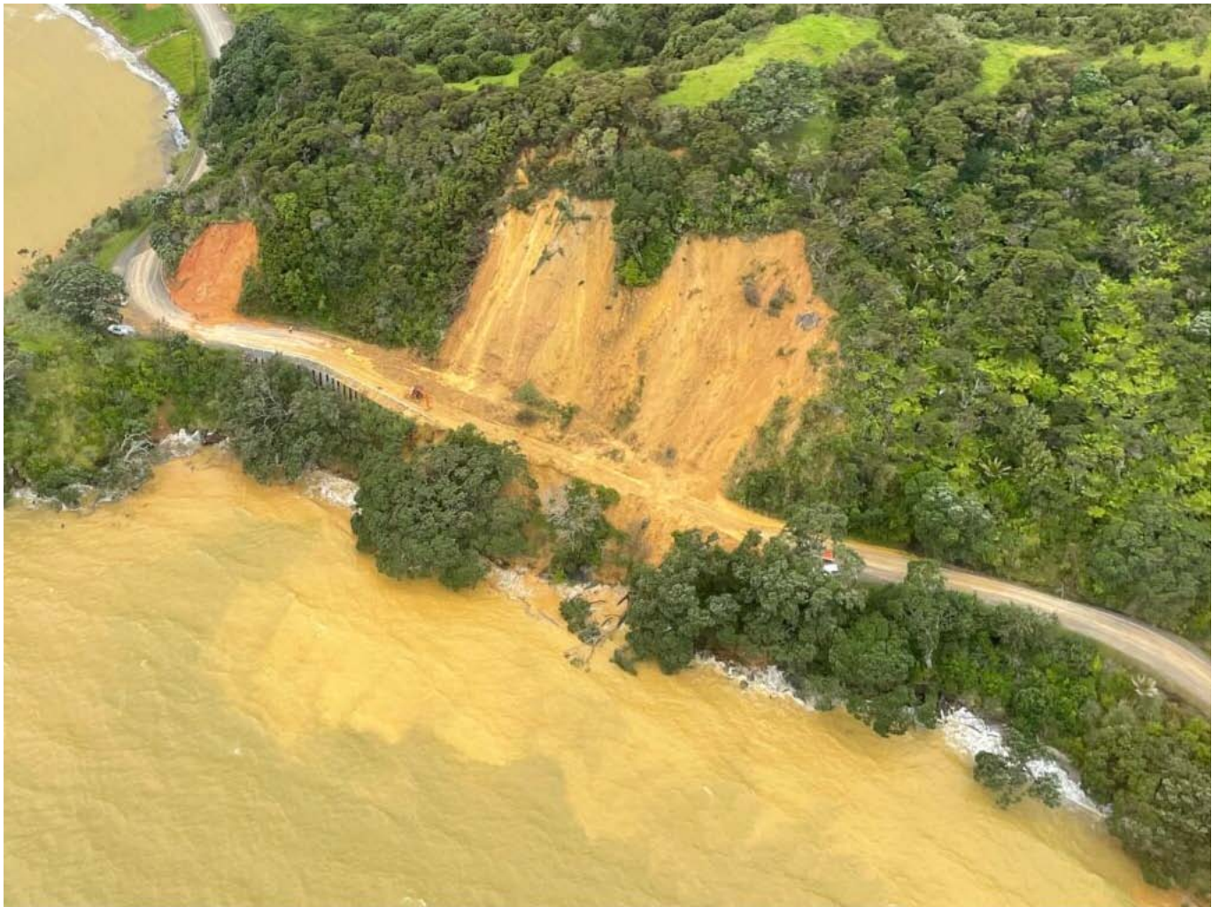
A major slip on the Thames Coast Road, State Highway 25. Photo: Thames-Coromandel District Council.
