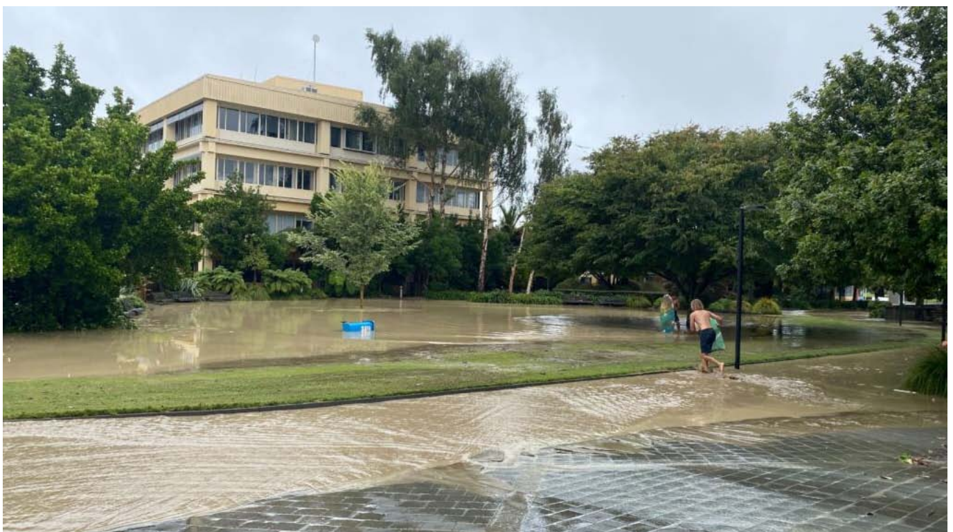
Eastern Institute of Technology Hawke's Bay campus in Napier has been badly damaged by Cyclone Gabrielle. Photo:
