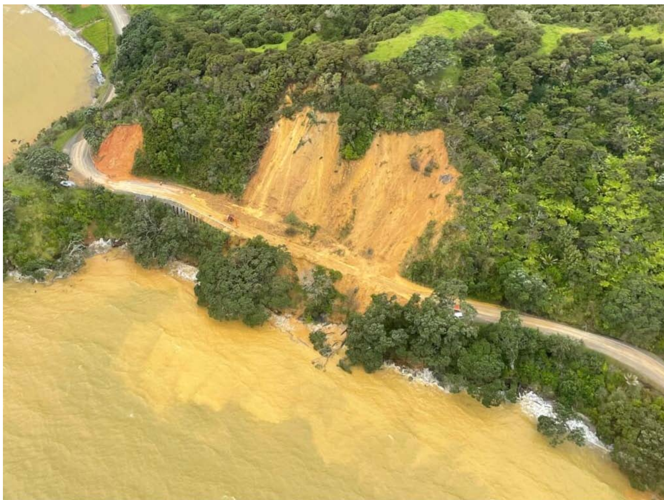
Road closures, including State Highway 25A from Tairua to Thames, will make it hard for nurses to get to work. Photo: Thames-Coromandel District Council.
