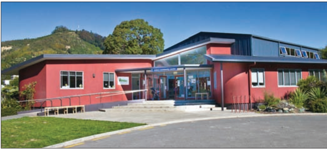
Victory Community Centre was opened in 2007.
