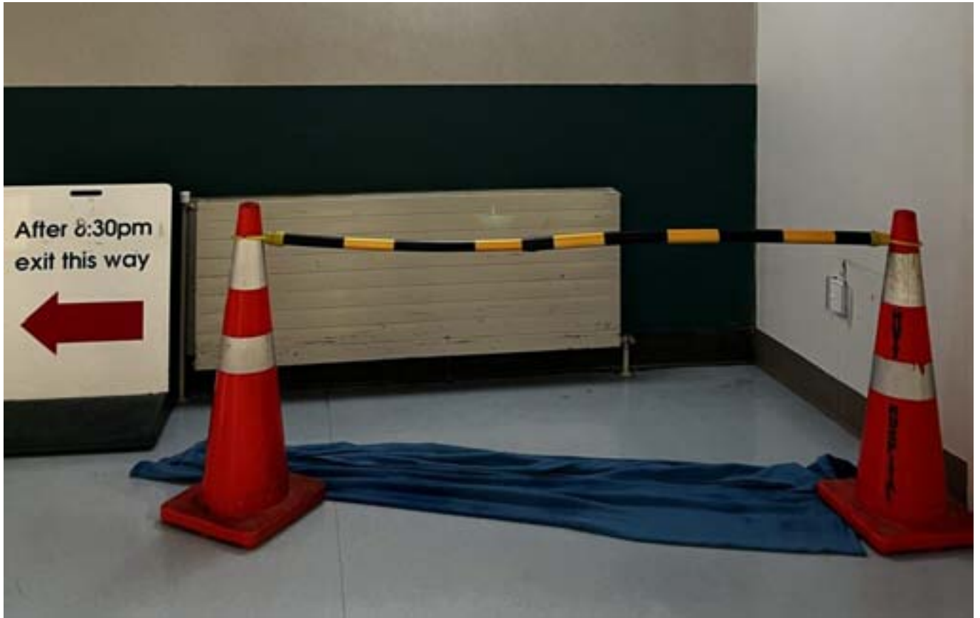
A no-go zone at Hutt Hospital following leaks.
